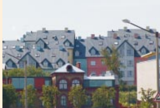
Development of area of Port of Tallinn
