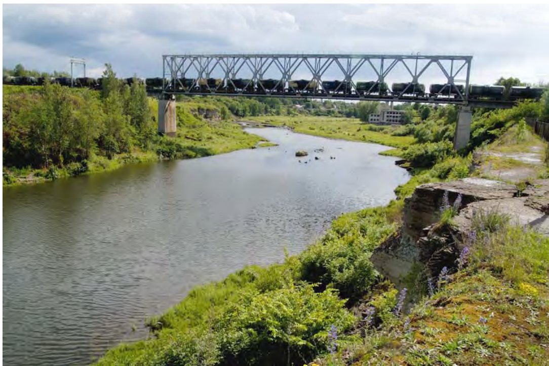
Foto 2. Raudteesild Eesti (paremal) ja Venemaa (vasakul) piiril ning Narva kanjon. Photo 2. The railway bridge on the border of Estonia (on the right side) and Russia (on the left side), and Narva Canyon.
