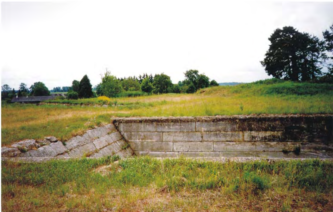
Foto 4.14. Loksa leiukohas on siloaugud Photo 4.14. In the quarry of Loksa
