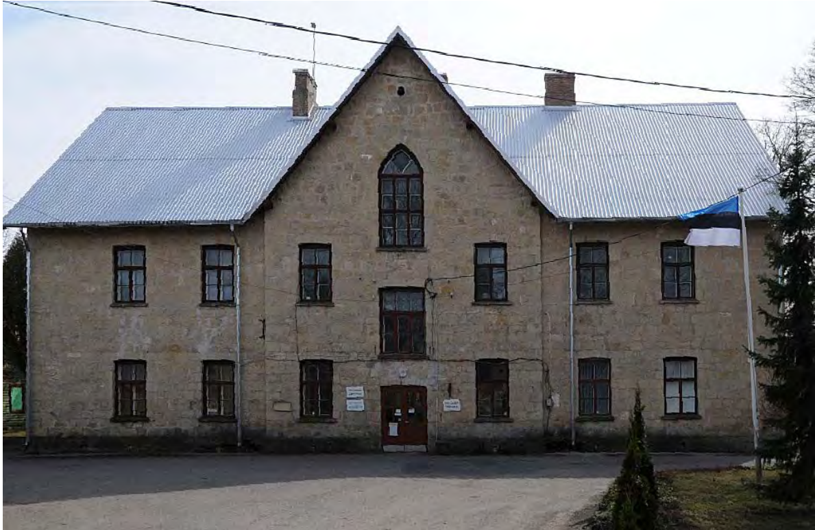
Foto 15. Endine Viru-Jaagupi vallamaja on ehitatud Inju dolokivist Photo 15. The former Viru-Jaagupi Parish House is build up of Inju dolomite
