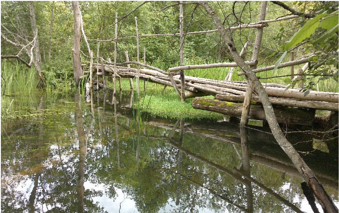
Foto 3.2. Purre Esna jõel Photo 3.2. The bridge over the Esna river
