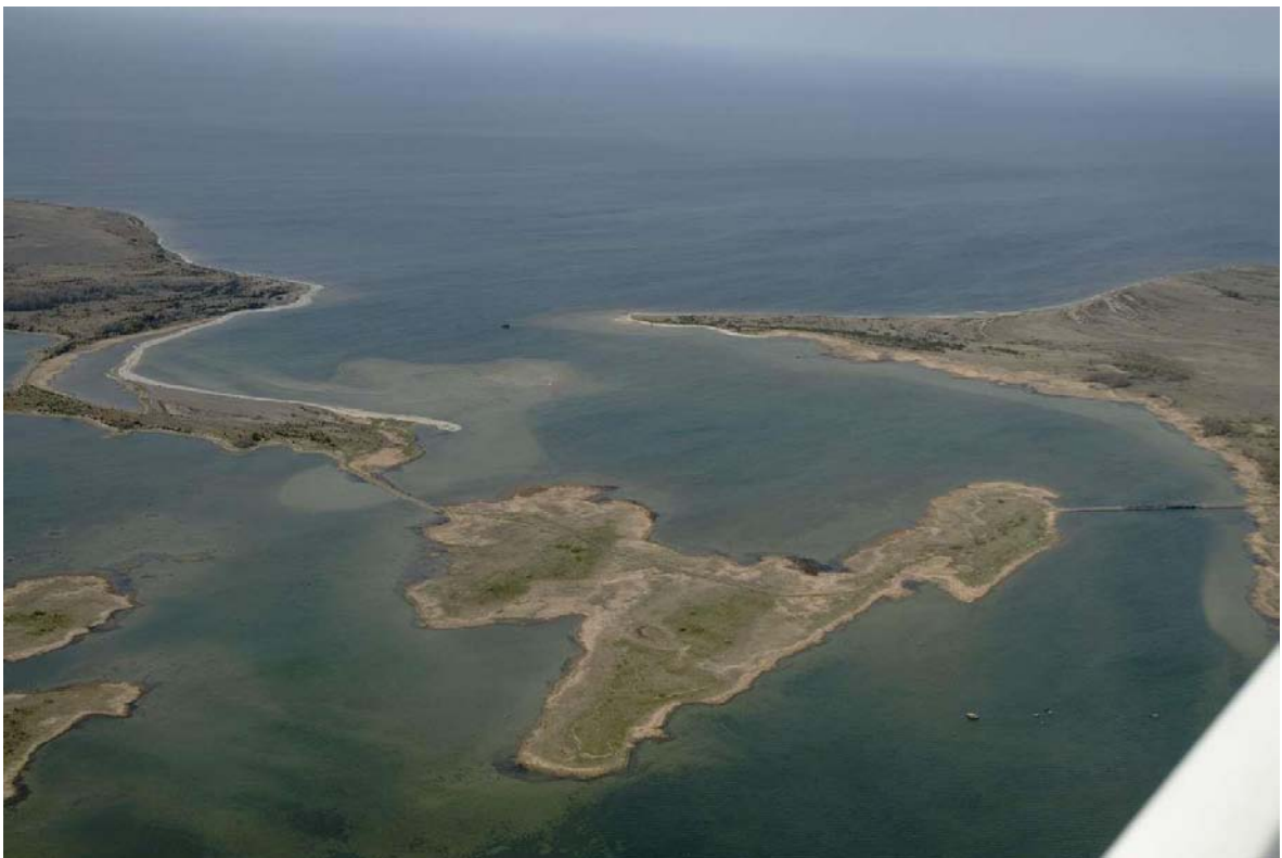
Foto 2. Õhuvaade Pakri saari ühendavale tammteele Photo 2. Aerial view to the causeway connecting Pakri islands
